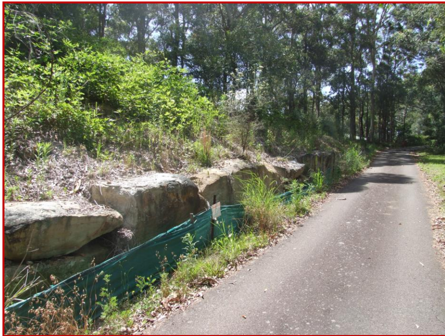
Figure 3-1-5. Photograph taken from a similar location as Figure 3-1-4, but looking west. Note the sandstone retaining wall. This was composed of both natural and artificial blocks, indicating both natural bedrock exposure and likely quarrying activities undertaken on the top of the ridge (just out of photograph in the upper left corner).
